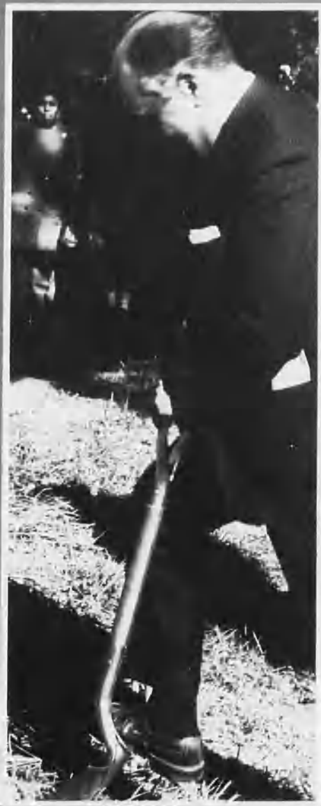
Breaking ground for the new.
